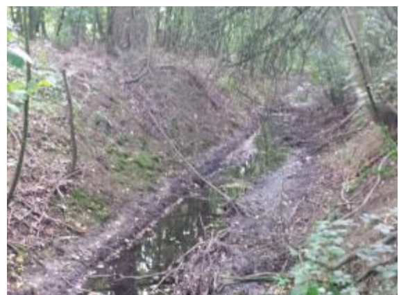
Photograph 4: Typical ditch section which flows east through a small area of broad-leaved woodland.
